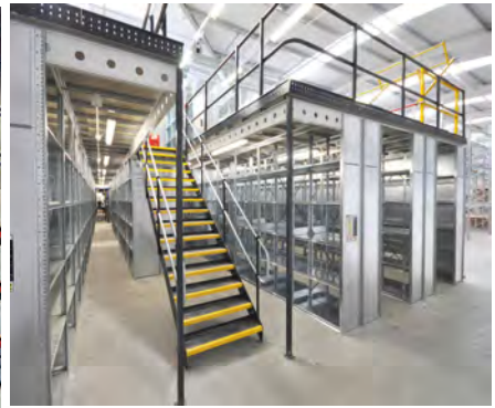
If walkways are placed, the height of the warehouse is visibility optimised.
